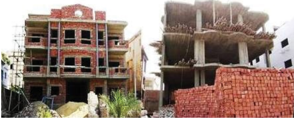
Figure 2. Load-bearing guard walls and structural buildings in New Cairo
